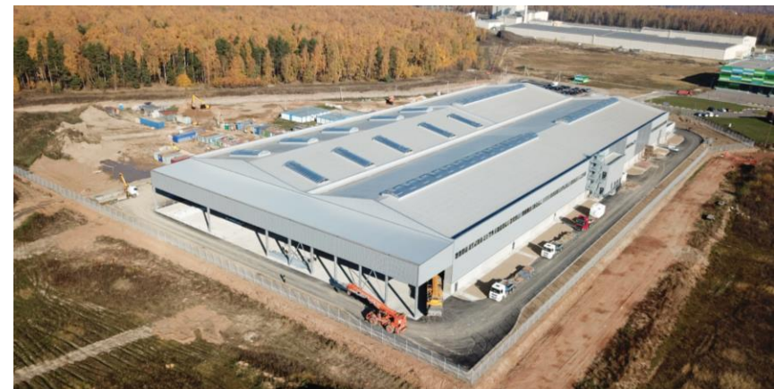
Plant Stupino under construction
