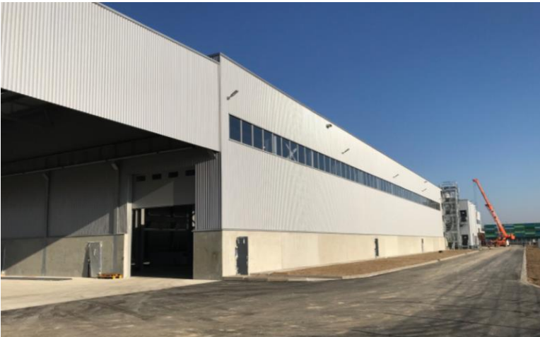
Loading roof (left)
