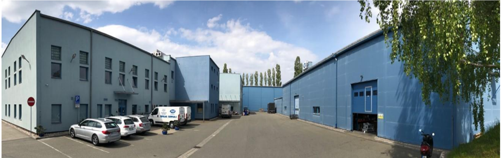
PZP Plant Dobré CZ
