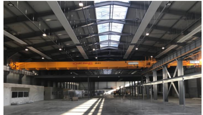
New radiant panel in Kermi plant RU (1,2 km)
