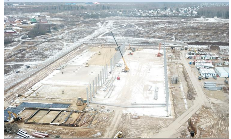
Site construction December 2017
