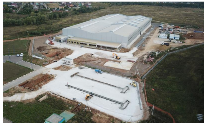
Site construction August 2018
