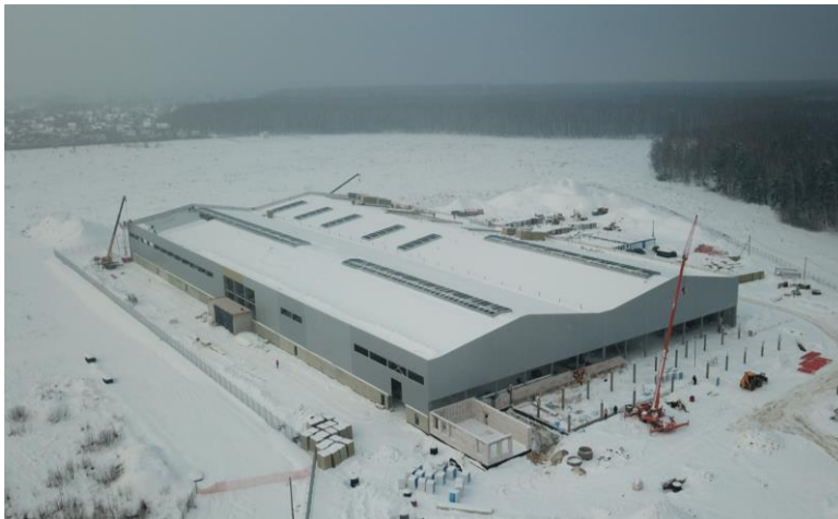
Site construction March 2018
