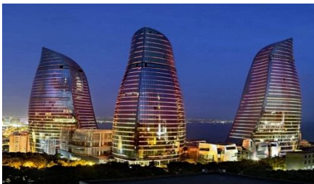
Flame Towers, Baku Fan Coils
