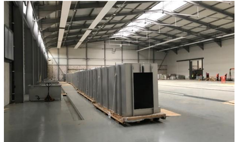
Building for paint shop – supplier Eisenmann started delivery
