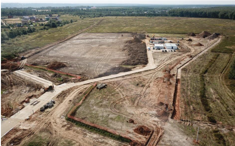
Site construction September 2017
