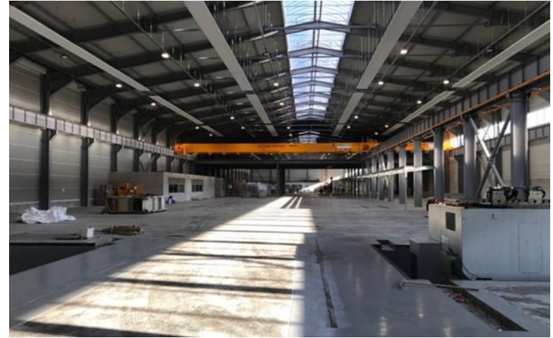
Building for raw production, ready for machine installation
