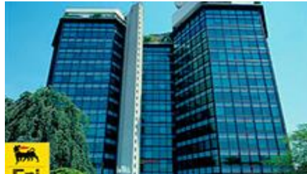
ENI Servici S.p.A. Headquarter Fan Coils
