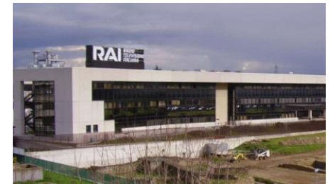
RAI Studios Rome Heat Recovery
