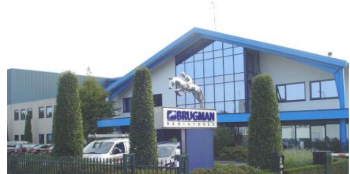
Brugman Plant Tubbergen, NL
