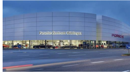
Porsche Center Böblingen Radiant Panels
