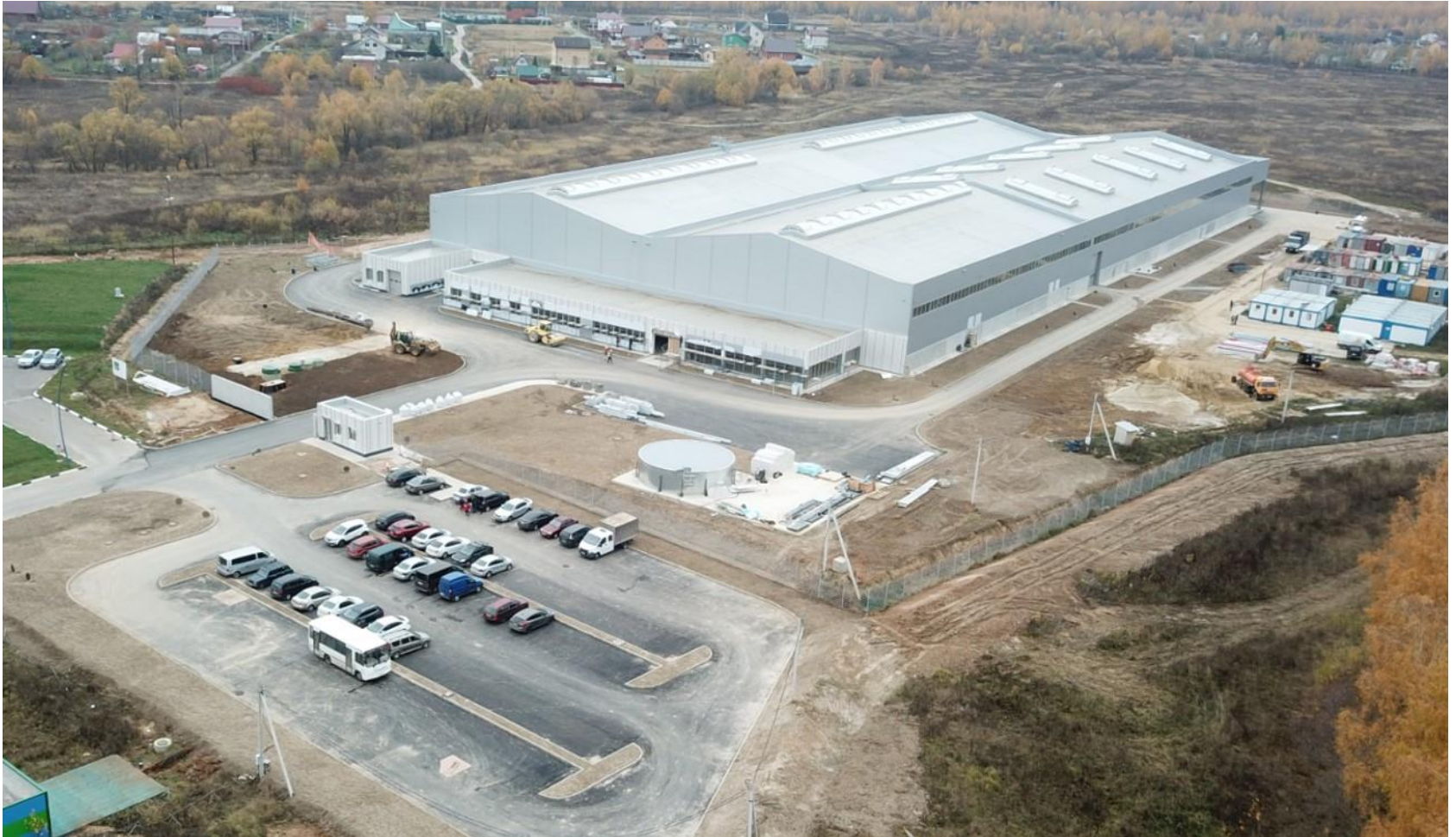
Kermi Plant Stupino, RU (under construction, 23.10.2018)
