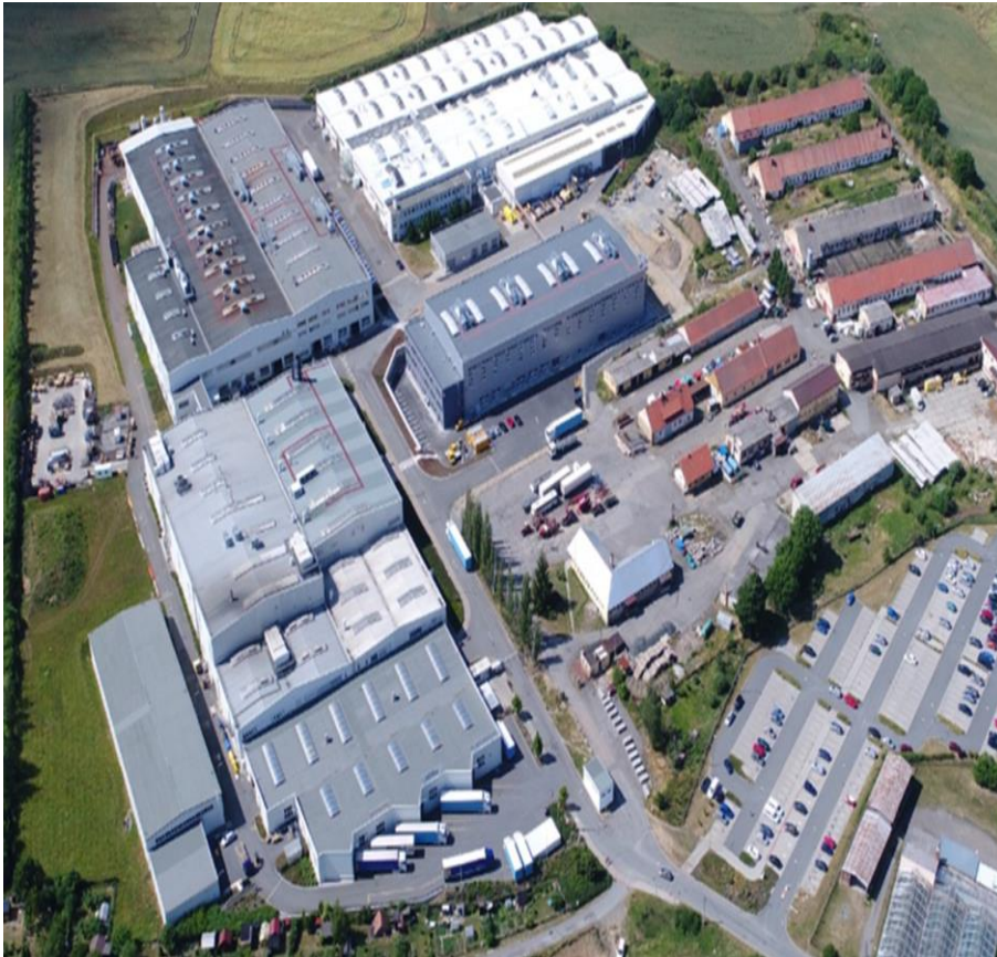
Kermi Plant Stribro, CZ
