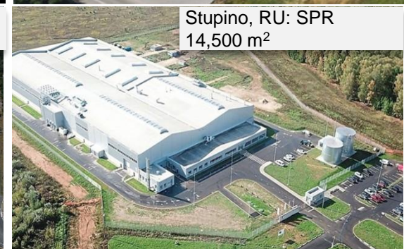
Corbetta, IT: ventilation 53,400 m 2
