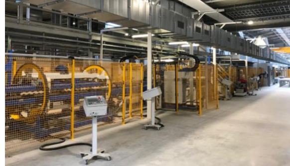
First of two welding lines
