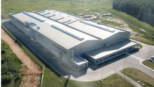
New plant – 15.000 m 2 covered area
